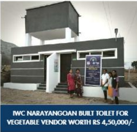
IWC NARAYANGOAN BUILT TOILET FOR VEGETABLE VENDOR WORTH RS 4,50,000/-
